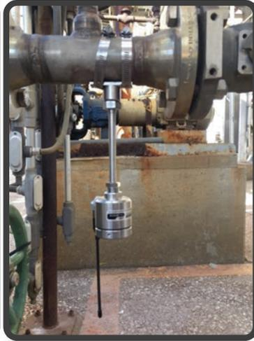
Dual-element unit installed using bands.
